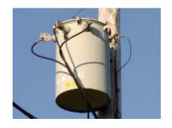
**Loose hardware** is a very common cause of power line noise along with faulty insulators, lightning arresters, or other hardware defects. Transformers are less likely the issue.
